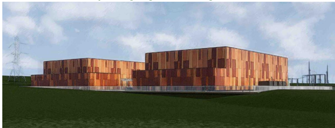
Plate 4.5 – Vertically arranged brown cladding
